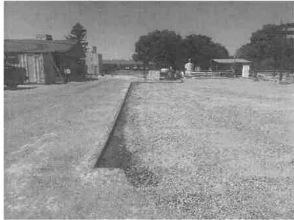
The Contractor cleans up sawcut edges of existing pavement.
