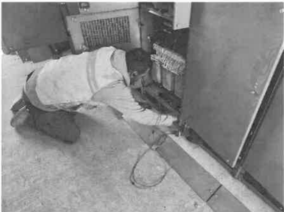
Central Sierra installs PLC and MCC anchors in electrical building.
