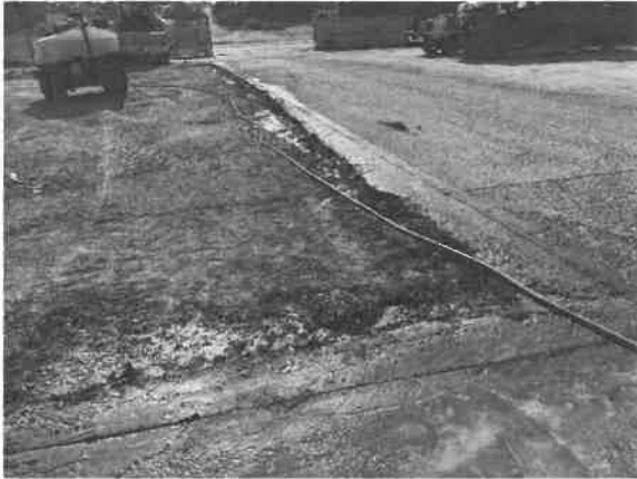
Contractor sawcuts edges of existing pavement to prepare for asphalt paving.
