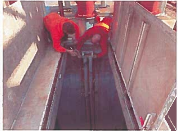
The Contractor grouts pedestals at slide rail anchors inside wet well
