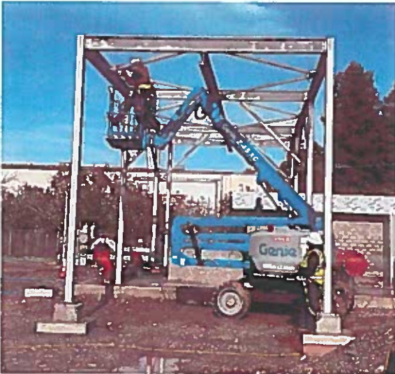
The Contractor welds the overhead crane structure.
