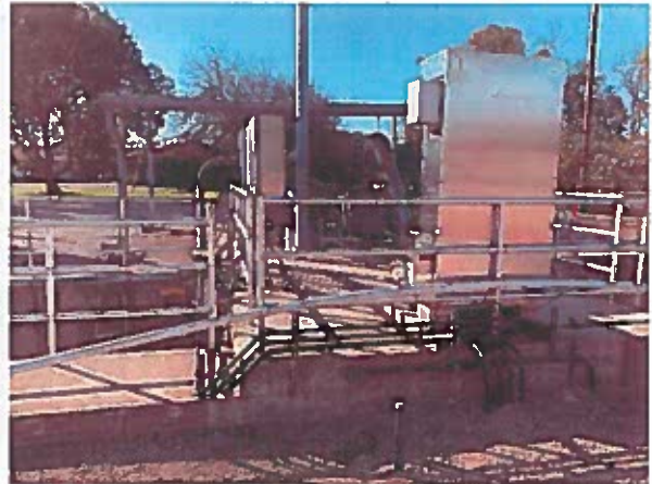
Central Sierra completes installation of conduits at the Influent Screening Facility.
