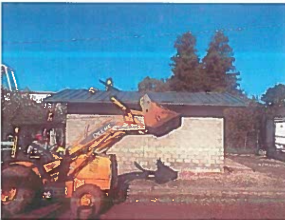
The Contractor completes metal roofing and flashing on the electrical building.
