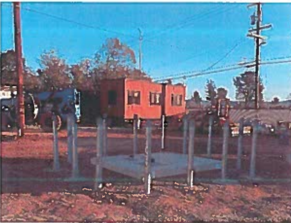
The Contractor sets bollards around the utility transformer pad.
