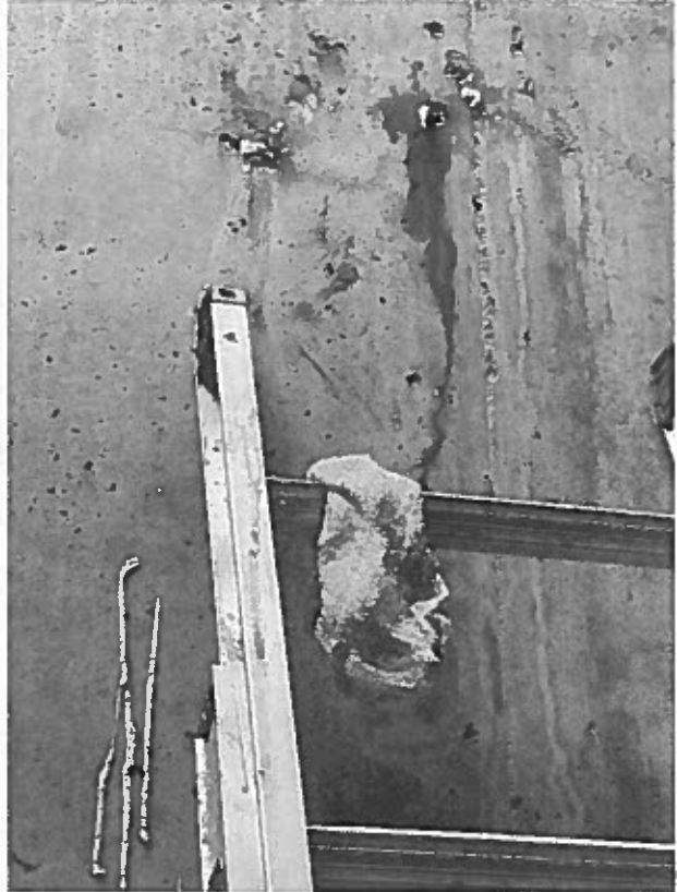
The Contractor sealed the leaks by applying SealBoss 1510 Water Stop Foam.
