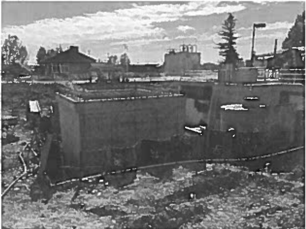
Outer formwork was removed from the wet well structure.
