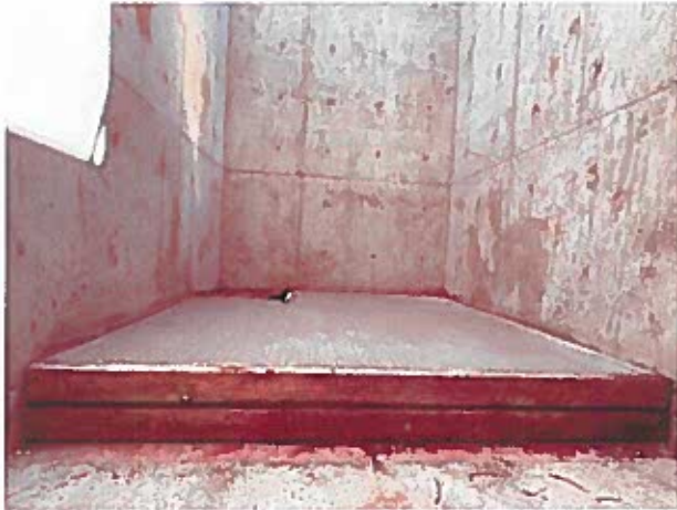
The platform in the bar screen structure was poured.
