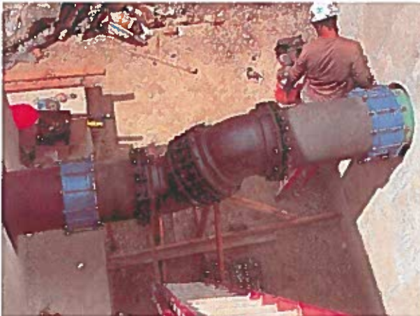
The Contractor installs 18" piping between Diversion Box 2 and the metering vault.
