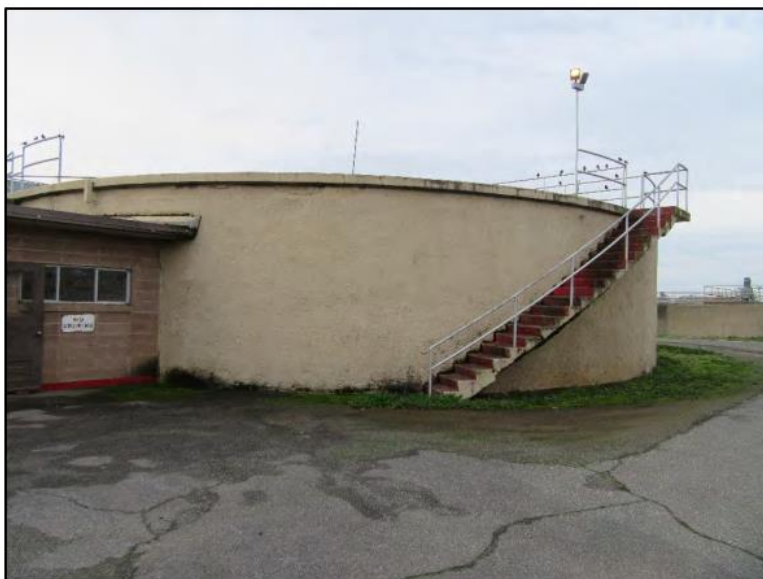
Figure 3-4. Southwest view of Resource OW-001 - 1950's tank located at the plant
