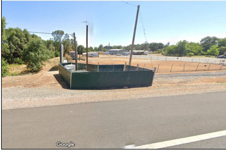
Figure 7 - View from south side of SR 162 looking southwest toward the pump station
