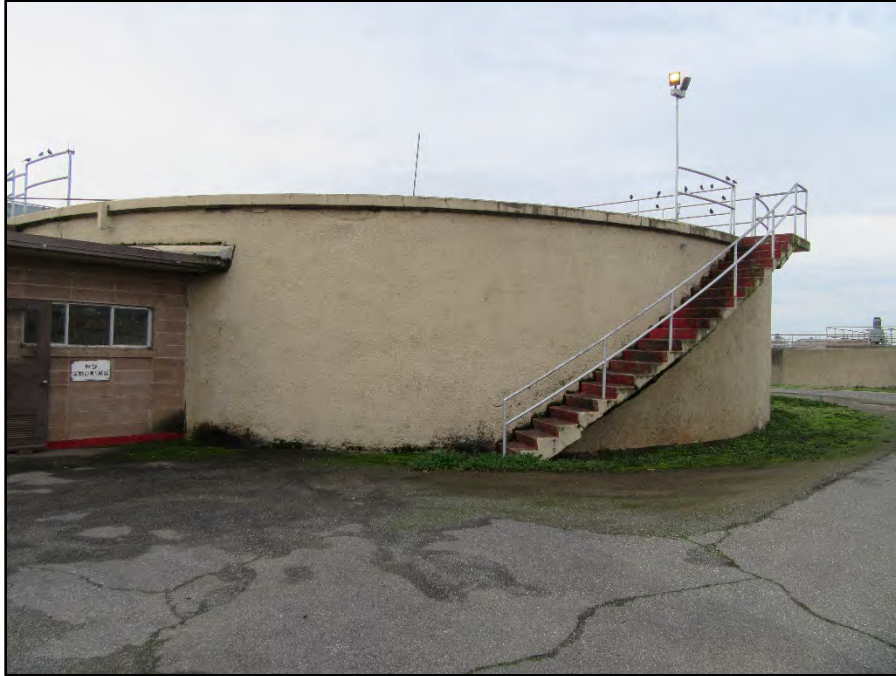
Figure 7. OW-001. 1950s tank located at the plant (view southwest) January 23, 2020.
